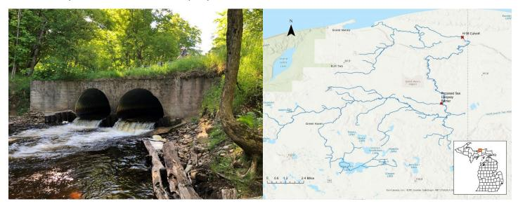
Replacing the H-58 culvert with a free span bridge and constructing a seasonal sea lamprey barrier further upstream in the watershed would provide for increased movement of non-jumping fish species further upstream and reduce the stream distance exposed to lampricides used to control invasive sea lamprey, while also addressing stream bank erosion. A free span bridge will provide all species access to an additional 20 miles of habitat year-round, and 115 miles seasonally.
