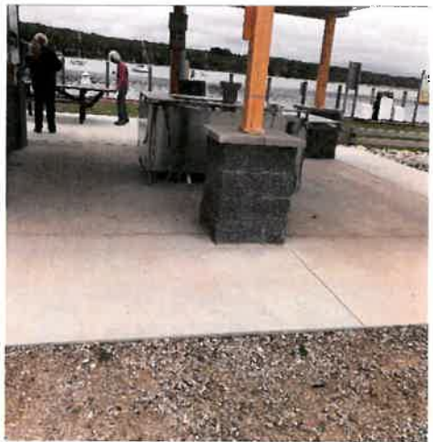
New accessible Fish Cleaning station
