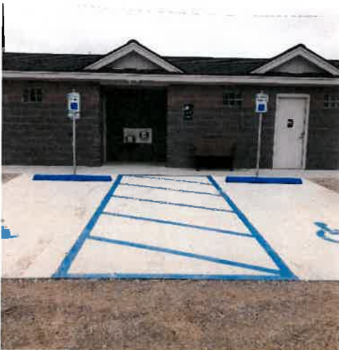
New Restrooms and Parking area
